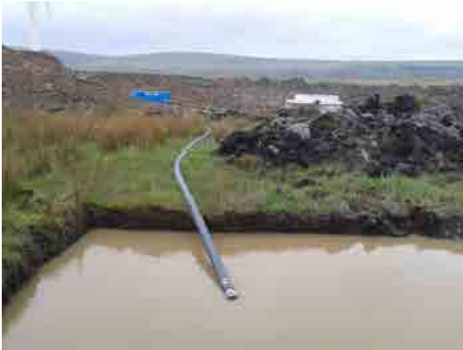
Plate 6: Typical 'Siltbuster' and settlement lagoon
