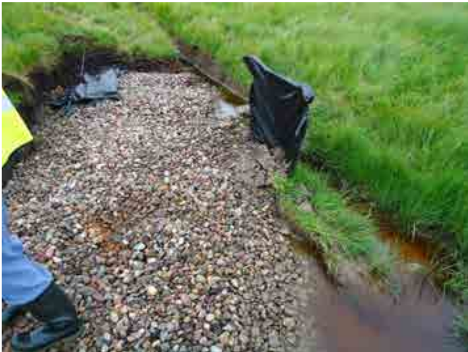
Plate 2: Typical silt traps
