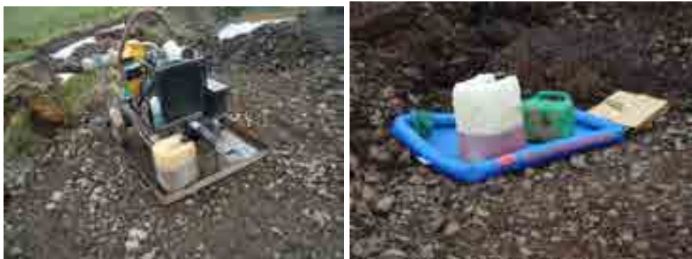
Plate 12: Examples of drip trays and bunds
