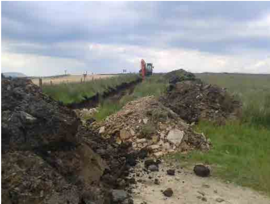
Plate 14: Typical overburden stockpile measures
