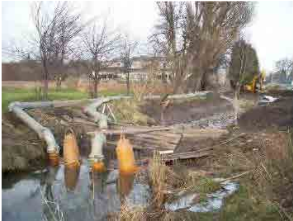
Plate 8: Full isolation - over pumping/siphon
