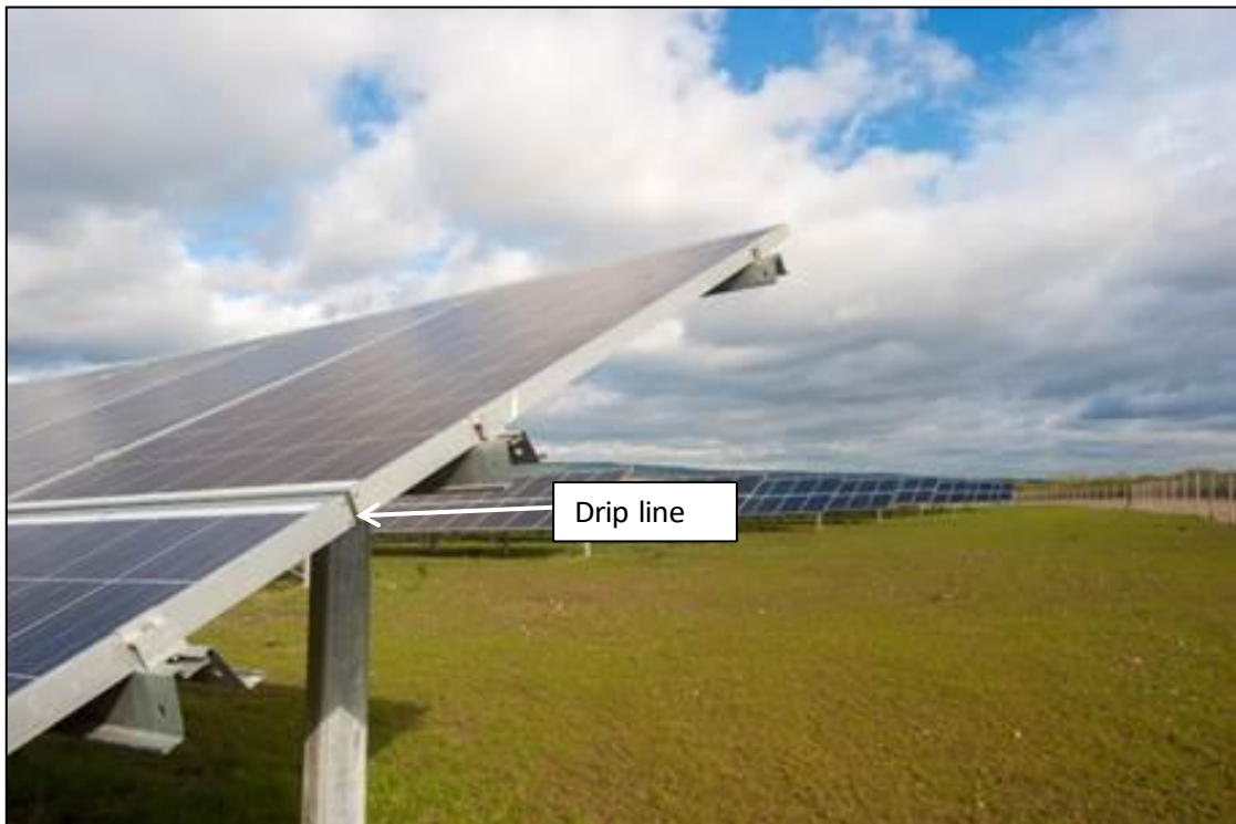
Plate 5: Typical PV racking system
