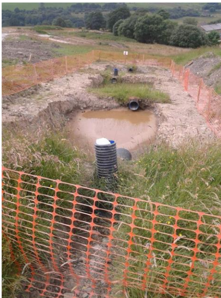
Plate 5: Typical lagoon and flocculent station
