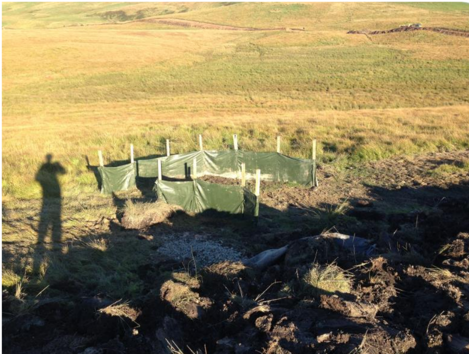
Plate 1: Typical silt fencing
