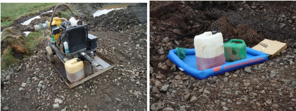
Plate 12: Examples of drip trays and bunds
