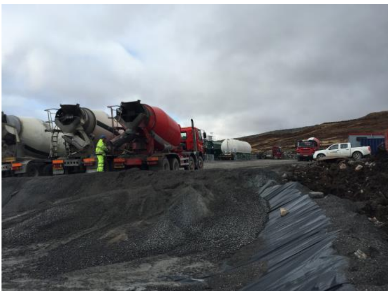
Plate 10: Typical concrete wash-out facility
