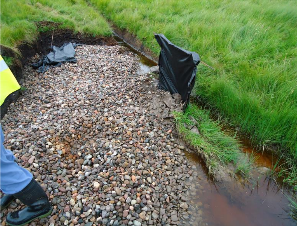
Plate 2: Typical silt traps
