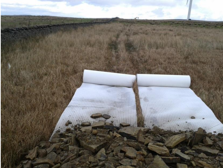
Plate 13: Semi-permeable geotextile layer
