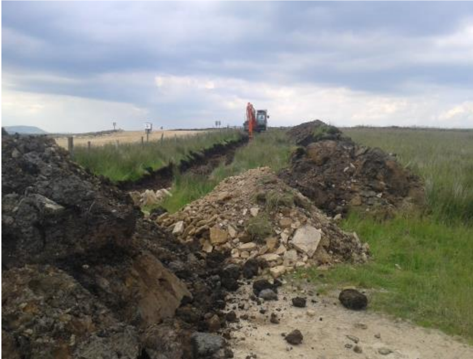
Plate 14: Typical overburden stockpile measures
