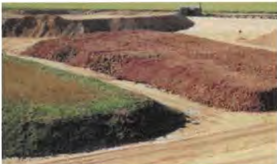
Clearly defined stockpiling of different soil materials
